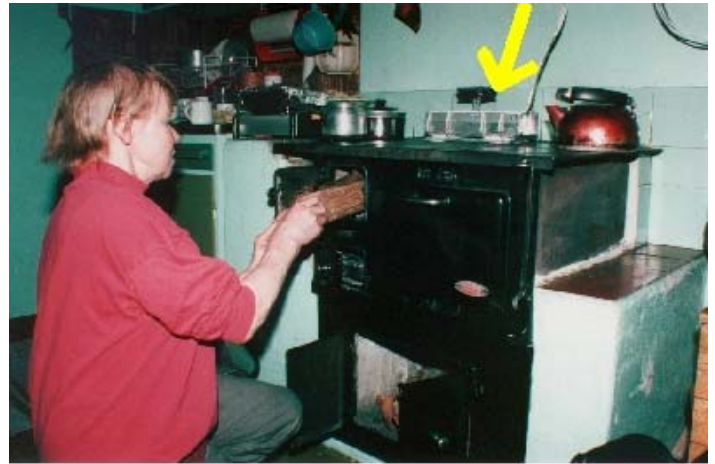
Figure4. Wood Stove With Generator at Left Rear
